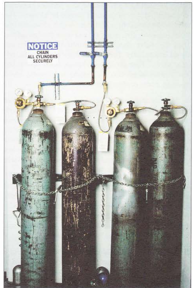
Figure 2.10—Inert Gas Cylinders Attached to Manifold System
