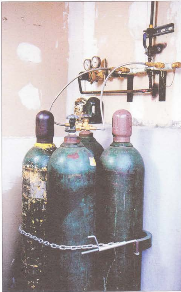
Figure 2.13—Oxygen Manifold System
