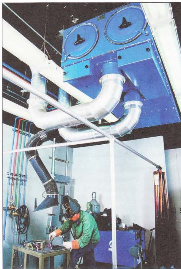
Figure 2.8—Movable Fume Extractor Positioned Near the Welding Arc
