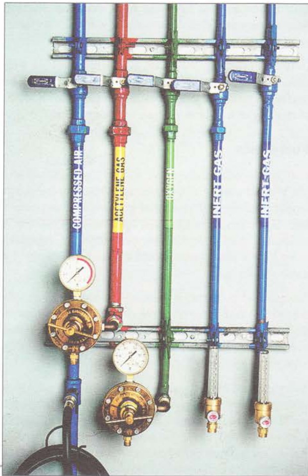
Figure 2.11—Acetylene and Oxygen Regulators and Inert Gas Flowmeters
